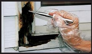
To strengthen the wood, apply LiquidWood with a brush, or pour directly on the surface. LiquidWood penetrates and hardens
