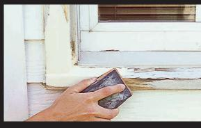
To rebuild missing pieces of wood and fill cracks and holes, apply WoodEpox. When hard, it can be sanded, stained, painted, and nailed
